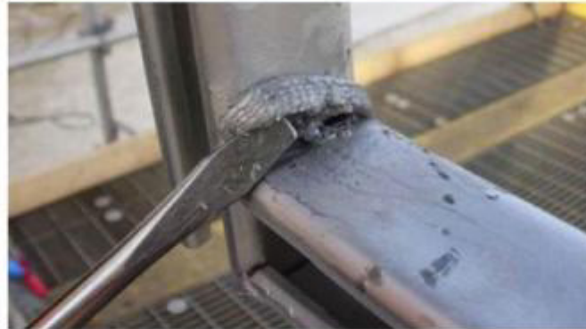
Photo 3 Silicon Welds
