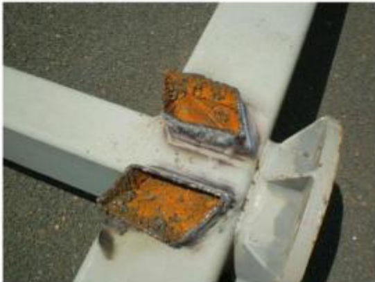
Photo 4 Diagonal chords on this bridge truss when cut were found to be filled with water. This is extremely unusual and is thought possibly to have been deliberate to build up the weight of the structure to have a mass within overall specification.
