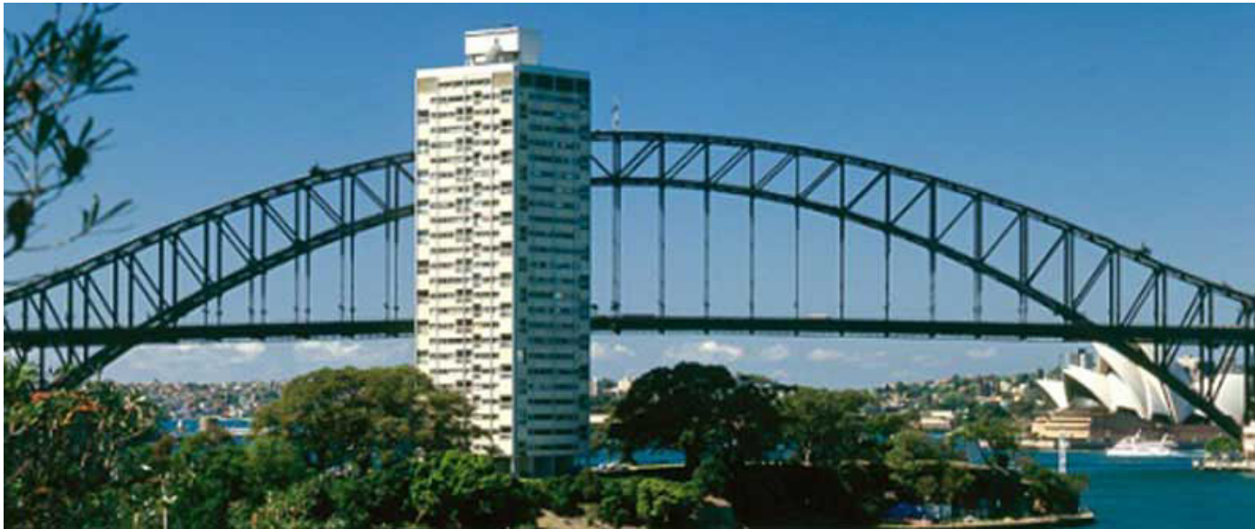
Blues Point Tower North Sydney 1962
